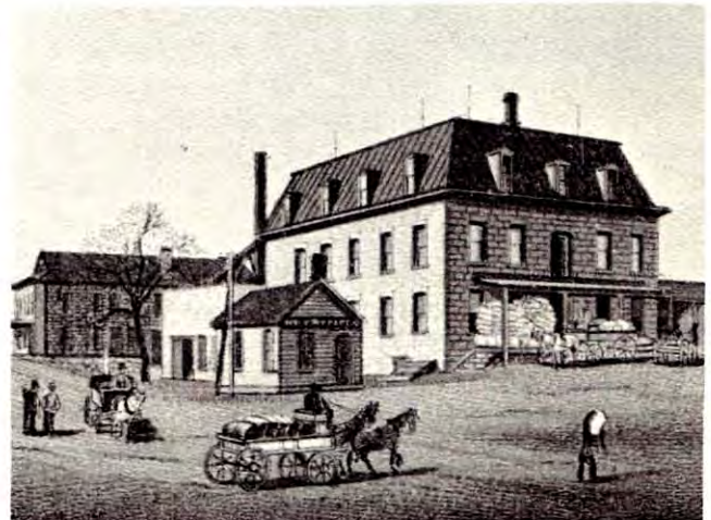
H. D. Crane and Company's Mill.
